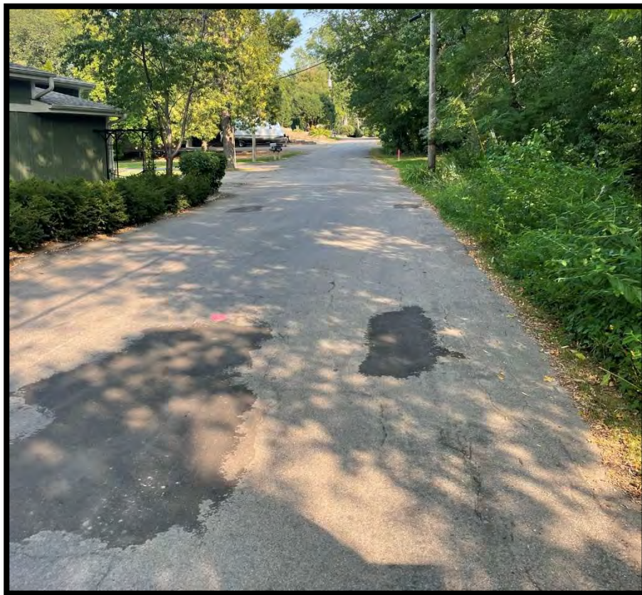
Photo 1. Brentwood Avenue looking east just before Bay Street.
