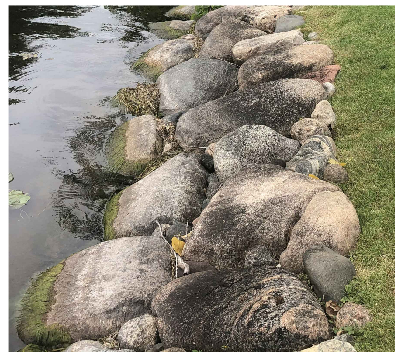
2 L3.2 RIP RAP ALTERNATE #1 PHOTO EXAMPLE
