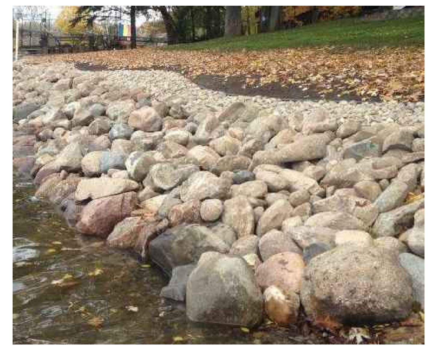
3 L3.2 RIP RAP ALTERNATE #2 PHOTO EXAMPLE
